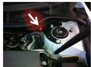
Distress (Green) Light Reset Switch
